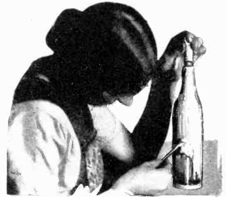
Gesso is spread over the surface of the bottle with a flat bit of wood. The wooden base and cork may be seen.
