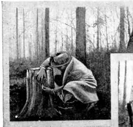
The tube, connected with a piece of ordinary blasting fuse, is placed in the hole in the oak stump and the hole is rammed loosely with rags. The fuse is lit, and WHAM! See what has happened to the stump!
