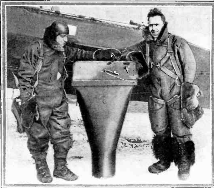
The photograph above demonstrates the size of the special airplane camera by comparison with the aviators standing beside it. This camera is designed to be used experimentally in photographing various portions of the terrain in the neighborhood of McCook Field, at Dayton, Ohio. The work is under the direction of Lieutenant G. W. Goddard, who is working in cooperation with the Eastman Kodak Company. The camera is probably the largest which has ever been assembled.
