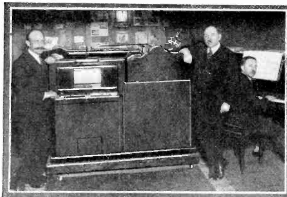
Two European engineers have perfected a device for mechanically reproducing, through the medium of player-rolls, the artistry of the finest violinists. The device is entirely pneumatic, and functions in a manner very similar to that of the automatic player piano. The results are said to be entirely satisfactory, even the bowing being perfect.
