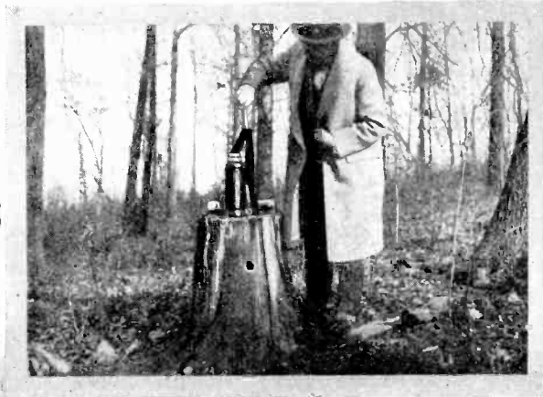
The stockings after being immersed in liquid oxygen contained in the thermos bottle are rammed into a short cardboard mailing tube closed at one end. Wooden pliers and a wooden ramrod are used to prevent "burning" the hands with the liquid. The tube is then stood on end and one half-a-cup of liquid oxygen poured into and over it, wetting the tube thoroughly.
