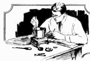
Here we see a home-study student checking up the electrical energy input and the output in heat of an electric stove. Practice must be coupled with theory.
