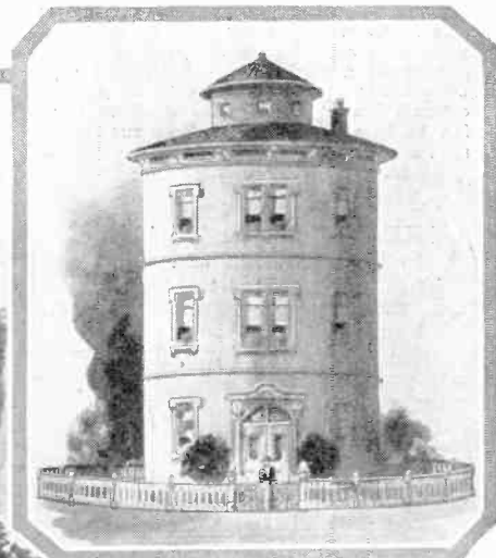
Cylindrical houses are being erected in Germany to solve the housing problem. The houses are of standardized construction, all sections being interchangeable. Standardization makes high-speed erection possible.
