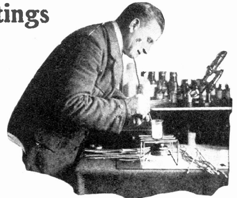
Paraffin is applied to the end of the slip where it has been previously carbonized.
