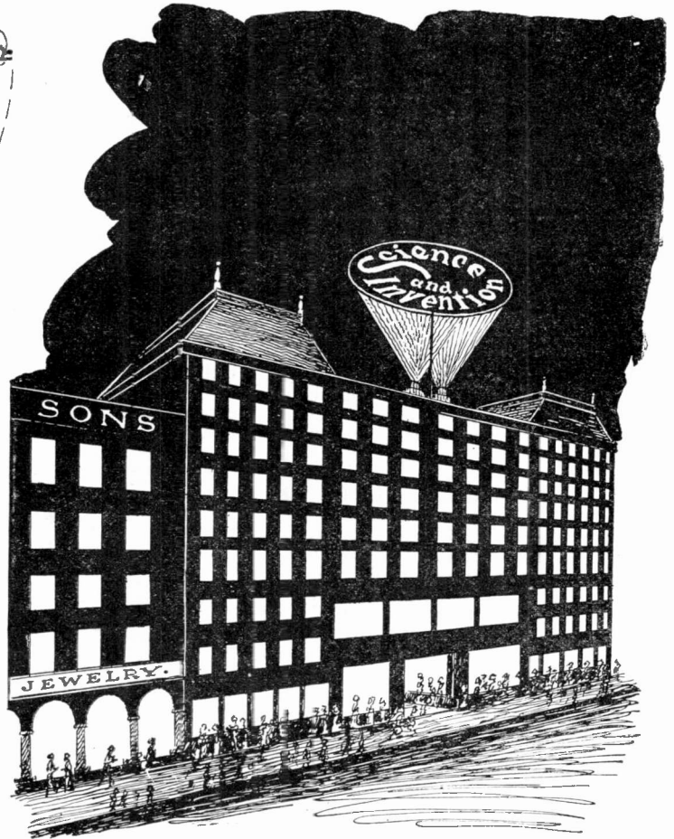
The illustration above shows the appearance of this rotary electric sign when in operation at night. The bulbs or reflectors on the outer edge of the circular frame provide the luminous border. If properly arranged, a sign of this nature is a most attractive night display.
