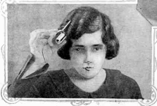
Another boon to milady's toilet is the small and compact curling iron illustrated in use below. The device is heated by means of a gasoline torch which is supplied with it and the prongs are then applied to the hair in the usual manner. In this way a young lady may keep her hair looking its best under all conditions. Despite its small size, this iron is said to be effective in every way and perfectly satisfactory in operation.
