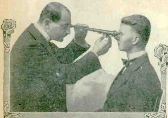
The instrument at the right is a foreign telescope only 23/4" long, which may be folded neatly into a box about the size of a match box. Its weight is about one-fifth of a pound, and it will magnify objects at short or great distances. Its field is at least three times larger than that of Galileian eight-power telescopes. —Dr. Albert Neuburger.
