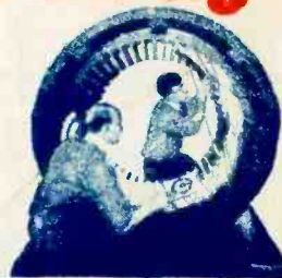
Student winding a Stator
