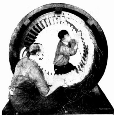
Student Winding a Stator
