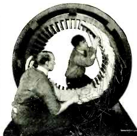
Student Winding a Stator
