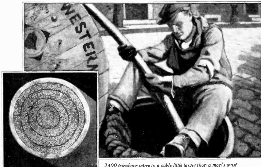
2400 telephone wires in a cable little larger than a man's wrist
