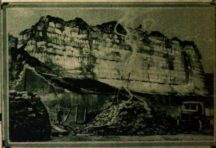
No, This Is Not an Iceberg from the North Pole, but One Made by Man. More Than 20,000 Blocks of Ice Are in This Land Iceberg, Comprising Over 6,000,000 Pounds of Ice. This Sight, Never Seen Before, Is in Covington, Ky., near Cincinnati, Where an Ice Plant Was Wrecked by an Ammonia Gas Explosion. The Force of the Explosion Was So Great That It Blew Away the Walls of the Building and Left the Ice Within Exposed to the Elements.
