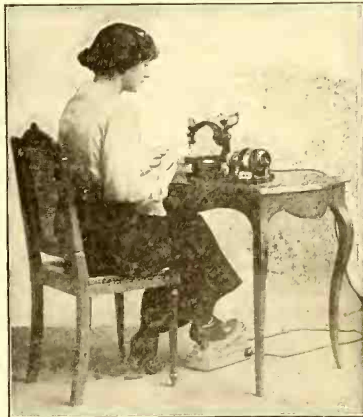
The Harder You Press on this Foot Rheostat the Faster the Motor Runs.
