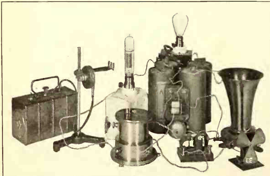
Fig. 12. Selenium Cell and Auxillary Apparatus for Laboratory and Lecture Demonstrations.
