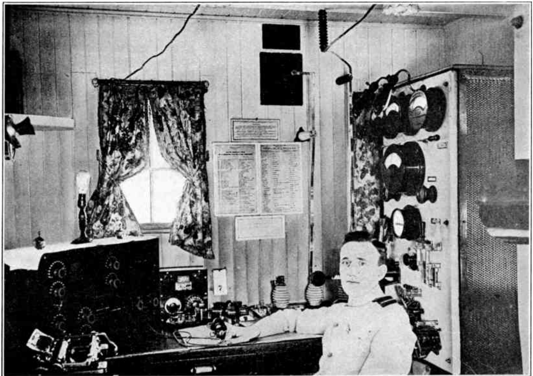
WIRELESS SPECIALTY APPARATUS installation on the United Fruit Co.'s Steamship Turrialba
