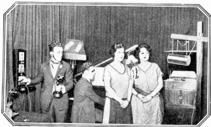
This picture shows how a duet is sent out from a broadcasting station. The small cylinder suspended from the frame at the right contains the transmitter. The man at the left is signaling the generator room, where the energy is controlled
