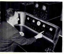
Master control board of NBC's television transmitter station, located on the 85th floor of the Empire State Building.
