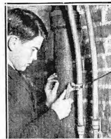
A Ground Clamp Simplifies the Ground Wire Problem.
