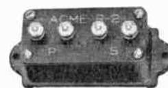
The Acme Radio frequency amplifying transformers, Type R-2, R-3, R-4.
