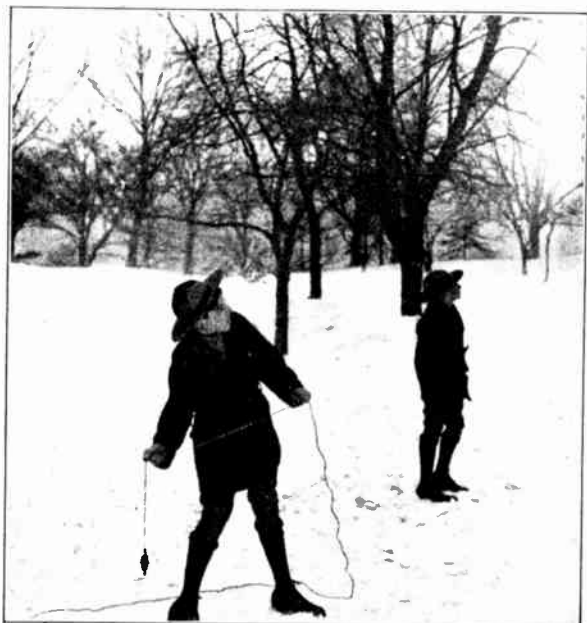
It is easy for the Boy Scout Signal Officer to erect a temporary aerial over a tree branch.
