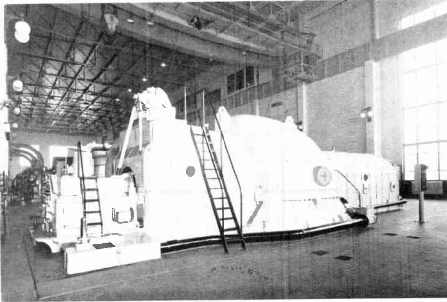
Fig. 2. The second 60,000-kw single-casing turbine-generator in Connors Creek Station of Detroit Edison Company
