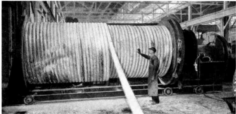
Fig. 51. Reel and picking device for handling long lengths of cable
