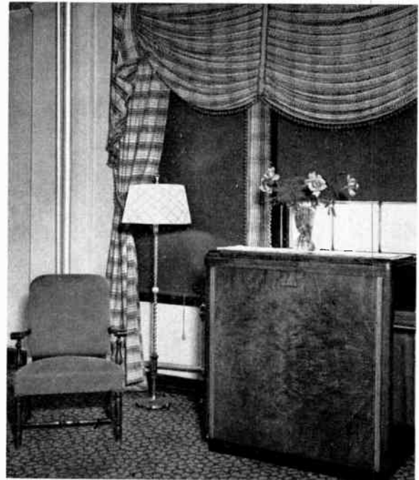
Fig. 113. Unit room air conditioner
