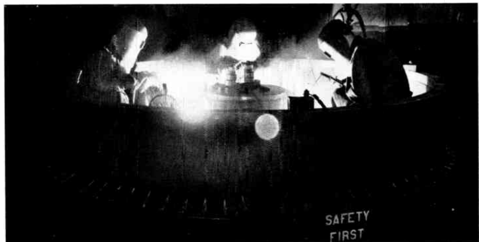
Fig. 70. Fabricating the low-speed gear of one of the new Gulf Oil Corporation tankers
