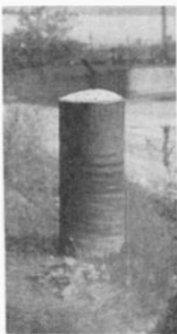
Snubbing post to lower heavy loads.
