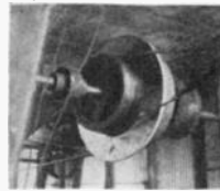
Separator for two close pulleys to prevent belts coming in contact.
