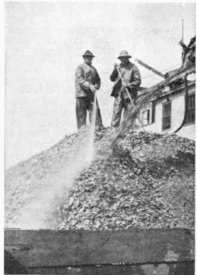
Shells coming from the revolving screens where they are washed and run into a barge.
