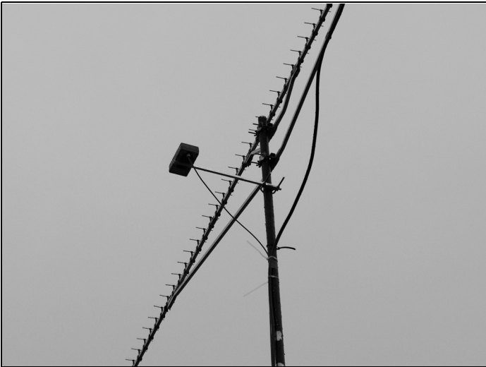
Fig 2: The Head Unit mounted on the mast.
