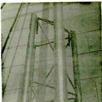
OUTSIDE VIEW OF TOP bracket gives another look at the hook arrangement.
