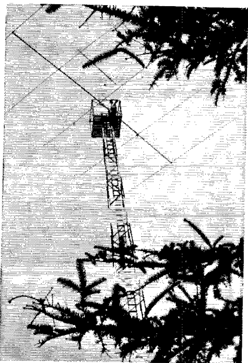
As he promised after the last test, I1BAF had a new antenna ready for this one. Mino used a 5-element wide-spaced array atop a home-built 100-foot tower. On the other bands: dipoles 80-foot up for 40 and 75, and 3 elements 60-foot up for 15 meters. Final results an outstanding two-thousand plus contacts.
