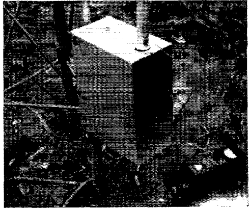
Fig. 4—Housing for matching capacitors at bottom end of the gamma rod.
