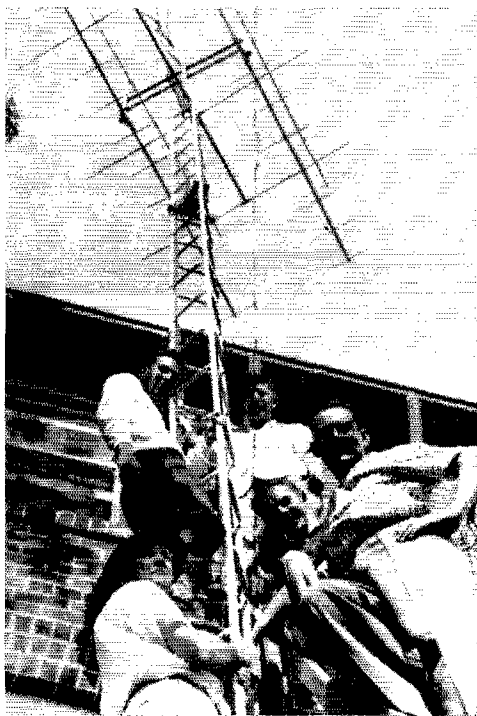
V.h.f. antenna going up in Canada prior to June contest. On top of tower: 3-element 6-meter beam, 16 elements for 2, 26 elements for 1 \frac{1}{4} . On tower—top left: John Ebersole, SWL; VE3BGB. Bottom left: VE3CWR, VE3BYU, VE3FBE.
