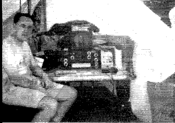
ZS6IF/8 and family scored 1358 QSOs with 62 countries early this year during a rugged week-long visit to Basutoland. The operating tent sheltered a 50-watt and modified HRO. A ground-plane did the radiating on 20 meters, a doublet on 15, and power was supplied by an 800-watt 110/220-volt gasoline unit. A view of the encampment shows the chow and sleeping tent at right, as well as some of the abundant animal-infested scenery. (Photo via W4PLL)
