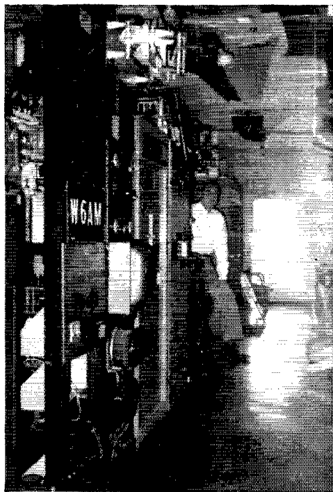
This photo of the W6AM final-amplifier bank complements views of Don's layout appearing on p. 74, November '57 QST. The kilowatt units, six in number, singly connect to a common power pack and modulator. All are deployed immediately behind the operating position (to left out of picture) so that most controls are within easy reach. (Photo via W8HCW)
