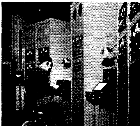
Inside a small AACCS station in the Far North.
