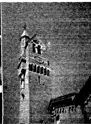
Antennas that bloom in the spring: L. to r. (1) The antenna of WKHF-16 dominates the city of Chicopee, Mass., from the belfry of the City Hall. The folded doublet shown has since been replaced with an extended double-Zepp, with improved results. (2) Tom Chapman, W1KK, and Joe Manning, W1GKY, putting the finishing touches on the Chicopee antenna. Their perch is 125 feet above ground. (3) Extended double-Zepp at WKHF-1 is more than 100 feet above ground, fed with 200 feet of open line. (4) Jess Richardson, W1CKJ (standing), and Howard Gourley, W1APP, rest up after erecting the new antenna for WKHF-1 atop the Hotel Kimball in Springfield.
