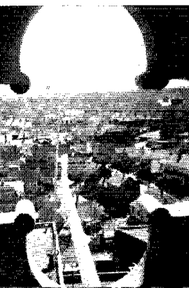
Antennas that bloom in the spring: L. to r. (1) The antenna of WKHF-16 dominates the city of Chicopee, Mass., from the belfry of the City Hall. The folded doublet shown has since been replaced with an extended double-Zepp, with improved results. (2) Tom Chapman, W1KK, and Joe Manning, W1GKY, putting the finishing touches on the Chicopee antenna. Their perch is 125 feet above ground. (3) Extended double-Zepp at WKHF-1 is more than 100 feet above ground, fed with 200 feet of open line. (4) Jess Richardson, W1CKJ (standing), and Howard Gourley, W1APP, rest up after erecting the new antenna for WKHF-1 atop the Hotel Kimball in Springfield.
