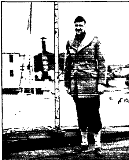
Capt. Vendley, 6AAE, member of the Third Army Training Inspection Team, on a visit to Ft. Clark, Texas, found this 55 beer-can vertical antenna on the roof of a cavalry signal section. Guyed at the middle with four wires, bottom fed, it has withstood several windstorms and is an excellent radiator. Capt. Vendley does not recommend the emptying of 55 cans at one time, however.
