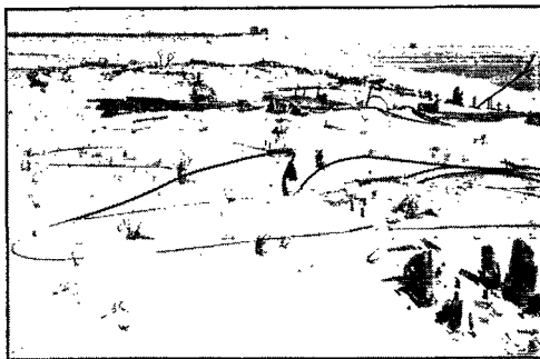
Anchor posts and pieces of guy wire of one of the masts can still be seen.
