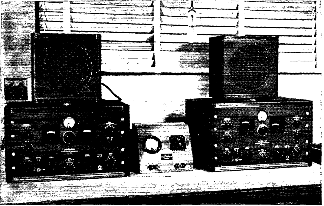
Diversity Receiving Installation at WABC
