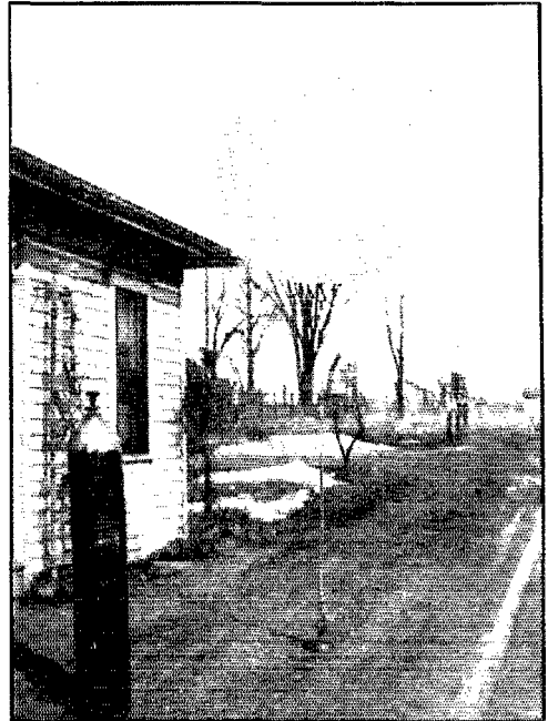
A balloon "sky hook" inflated and ready to take the antenna upstairs for a week or so. The hydrogen tank is in the left foreground.
