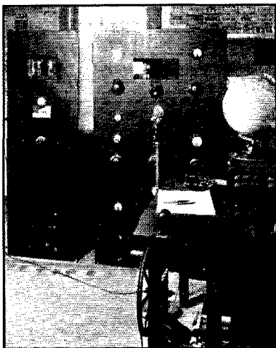
THE MODULATOR AND KILOWATT TRANSMITTER OF W3PC, PORT REPUBLIC, N. J.
