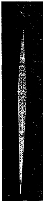
THE MAST AT WIDHT, BRISTOL RADIO CLUB, SOUTH MOUNTAIN, BRISTOL, CONN.
