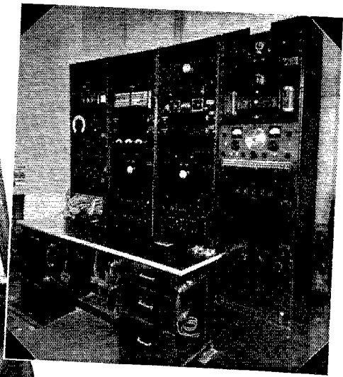
THE CONTROL BOARD OF WFBR, NBC station of Baltimore, Md., showing panel installation of 1938 Super Skyrider.
