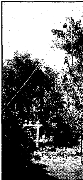
FIG. 6—THE TUNED-TOP VERTICAL ANTENNA INSTALLATION AT AMATEUR STATION W2ETH
