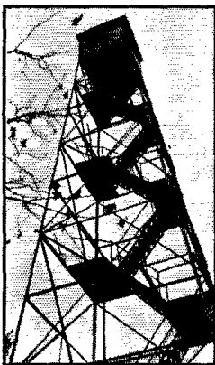
A TYPICAL SIXTY-FOOT OBSERVATION TOWER OF SIMILAR TYPE TO THOSE MADE AVAILABLE TO THE NEWJERSEY AMATEURS
