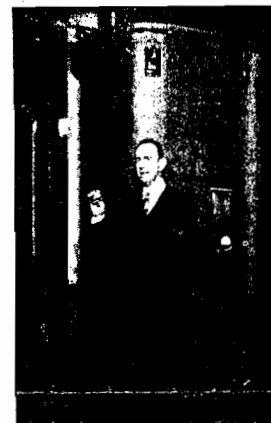
Here Powel Crosley, Jr. is holding in his hand one of the smallest audio transformers formerly in use for WLW. Behind him is seen a portion of the huge audio transformer used in connection with the 500,000 watt transmitter. It weighs over 35 tons and is, by far, the largest in the world.
