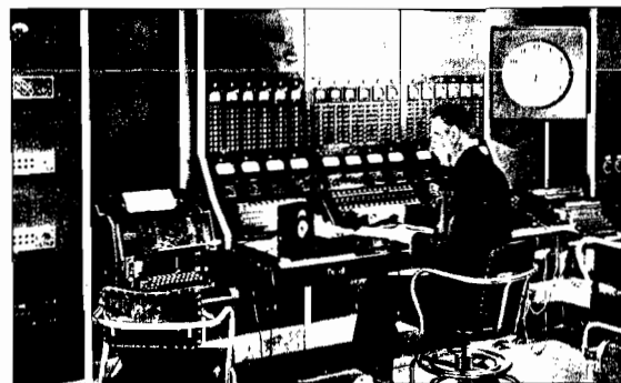
Master Control — This control center fed programming down a bank of phone lines to the transmitter site. During 500 kw years, WLW program listings appeared in up to seventy-six newspapers from Texas to Connecticut. Programs were routed to WLW, WSAI, WBAI, the "New York Line" and various national networks.
