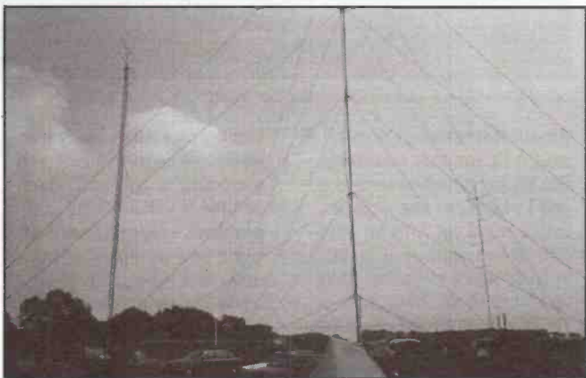
Windmill CG in VHF FD 1991. The 15m rotatable mast for 4m has its base in the middle of the tent and rotation is by the 'armstrong' method. The 30m tower to the left supports two 70cm yagis and was put up using a gin pole made of 12m of tower section, and a winch mounted on a Land Rover.
