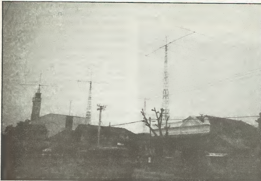
Fig. 5. YBOWR's antennas: left to right, 3 element on 40m, 6 element on 20m (with VHF/UHF antennas above), KT34XA 6 element tri-bander, and a 4 element 80m beam.
