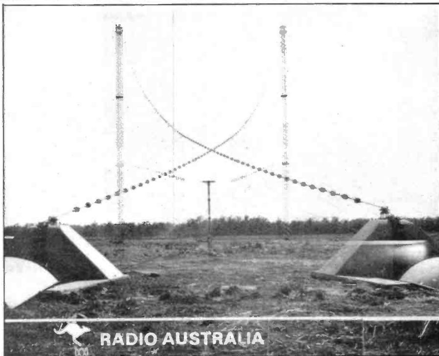
A QSL card from Radio Australia illustrating one of their log periodic transmitting antennas.
