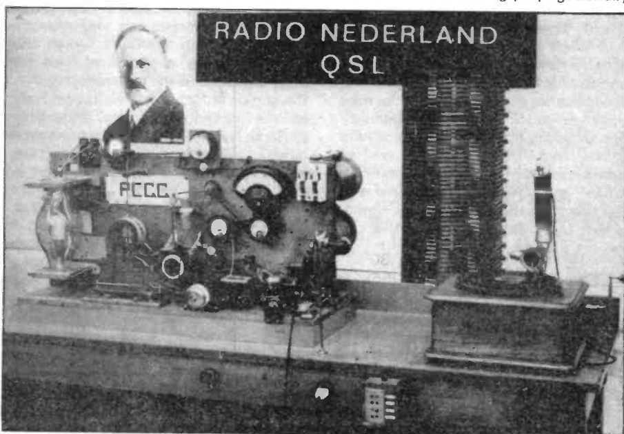
The first broadcasts from the Netherlands were as long ago as 1919; this is the original transmitter which used the callsign PCGG and which is now on show in the Posts Museum in the Hague.
