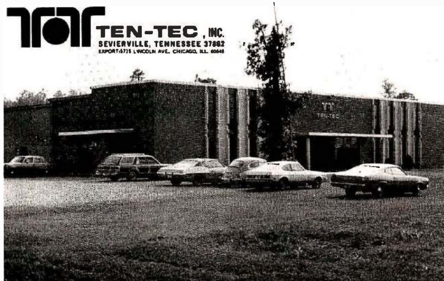
“Here’s a photograph I took of the Ten-Tec plant in 1978. It doesn’t show the entire building, but it is a neat, modern facility. Their products are neat and modern, too. No, I don’t work for Ten-Tec — I’m a pharmacist!” KA3BGP.
