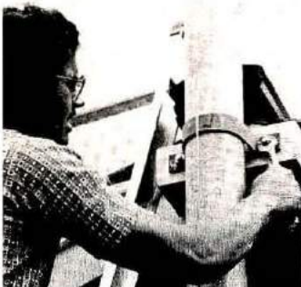
Mounting the House Bracket
