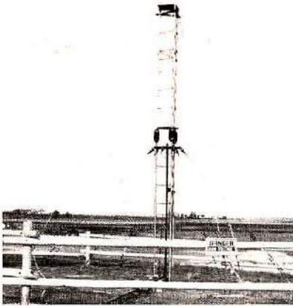
The 25-MHz dipole antenna near the WWV building. It is center fed by means of the 3-1/8 inch (8cm) transmission line you can see in the left foreground (photo courtesy US Department of Commerce).
