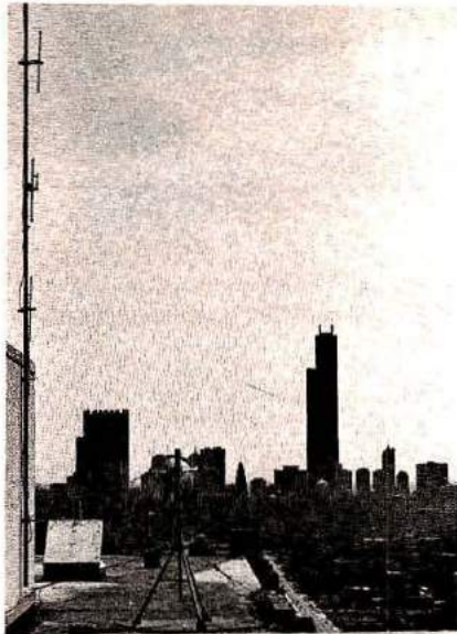
Tall buildings in large cities collect their share of repeater equipment. Here a Cushcraft 4-dipole antenna is part of the Chicago FM Club's 220-MHz repeater. The skyline to the south of the repeater site includes the Sears Tower, Standard Oil Company building, First National Bank, and others among the tallest buildings in the city (photo courtesy Chicago FM Club).
