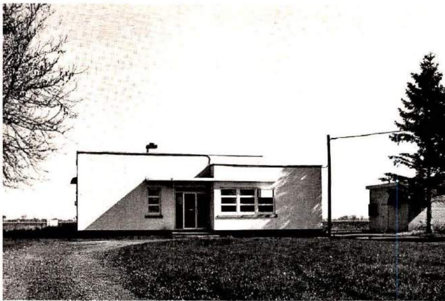
The main building, left, and generator building, right, for time and frequency station CHU, in Canada (photo courtesy Canadian National Research Council).
