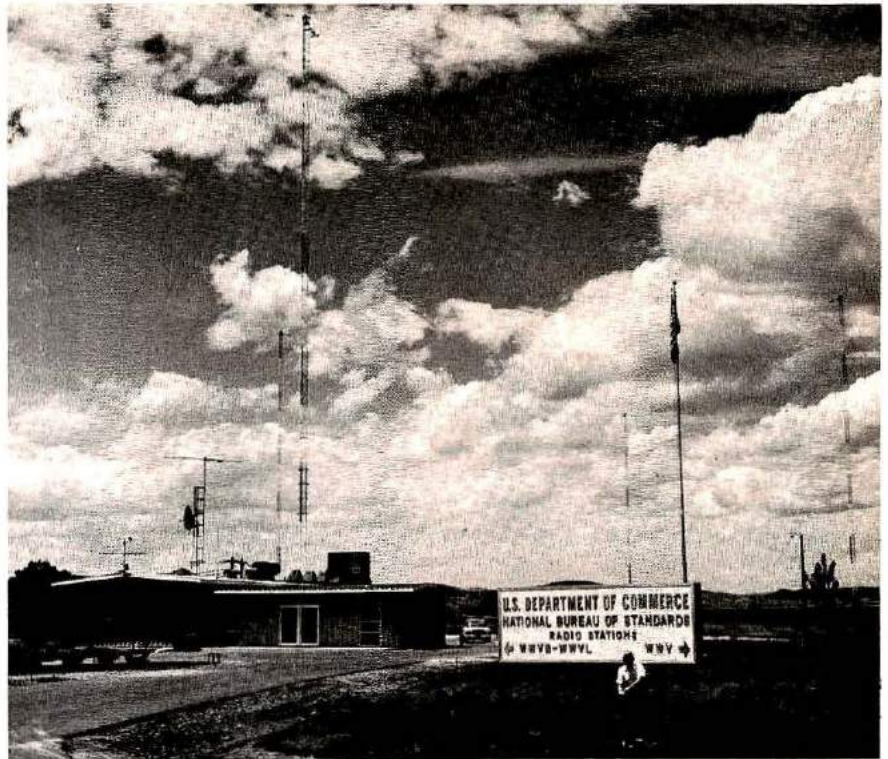
This building is where the low-frequency transmitters, for stations WWVB and WWVL, are located. The towers support large wire antennas, but the largest is out of the photograph to the left. Prospective visitors should check with the US Department of Commerce in Boulder, Colorado, about the availability of tours at the WWV transmitting site (photo courtesy US Department of Commerce).
