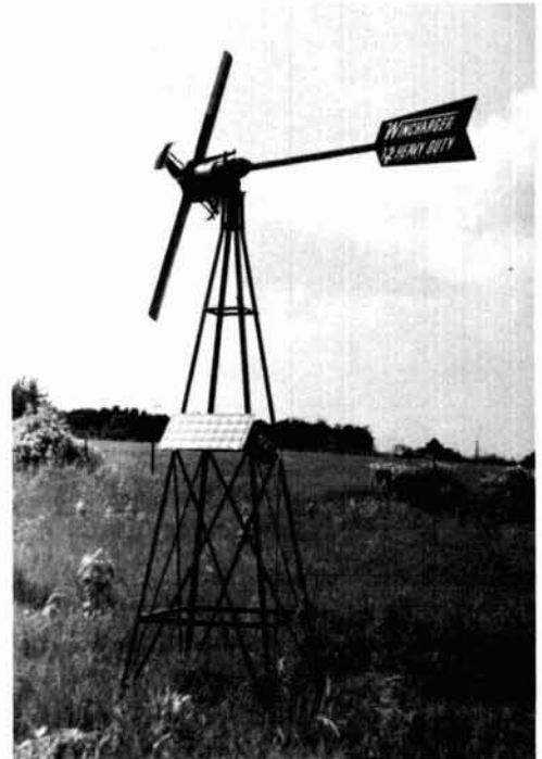
fig. 9. Winco generator and Solarex panel installation at W3FQJ.
