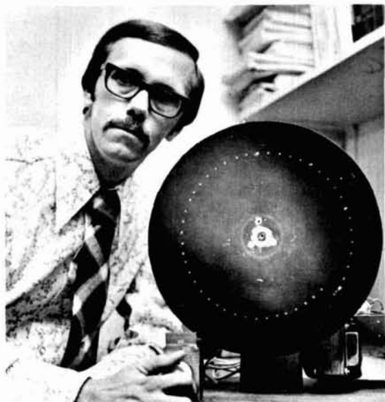
K4TWJ and the Nipkow disc he built to reactivate 1925-style TV.
