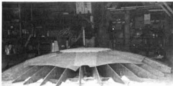
Partially finished pattern.
