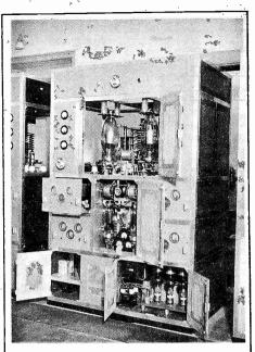
2RO PANEL NO.1 Housing The 49.3 Meter Transmitter
